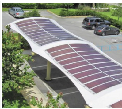
Flexible Organic Solar PV on Curved Parking Lot Carports and on a "Solar Tent"
