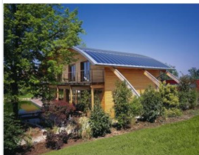
Solar Rolls Attached to Curved Roof
