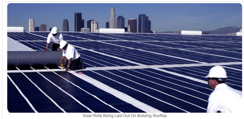
Solar Rolls Being Laid Out On Building Rooftop
