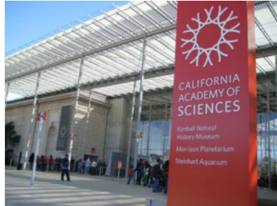
Solar Roof at California Academy of Sciences, San Francisco
