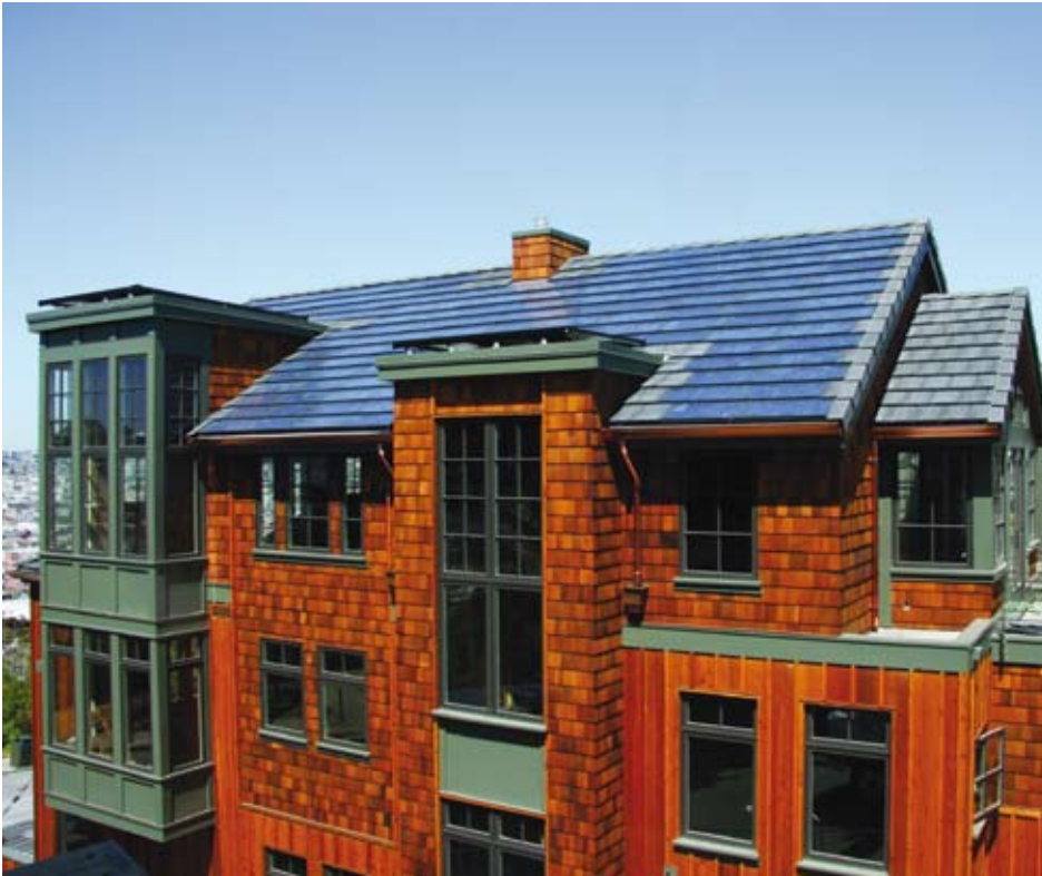
This house features the Eagle Solar Roof with SolarBlend, a system of polycrystalline silicon tiles from Suntech Power.
